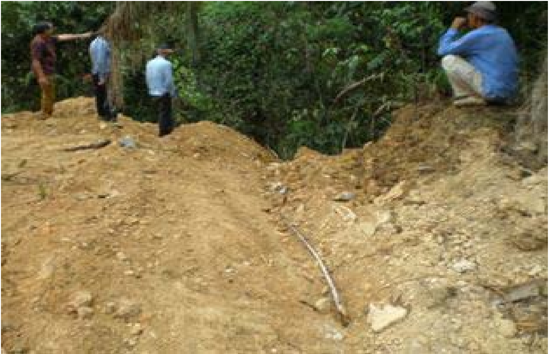
Drain flow to Belaga river
